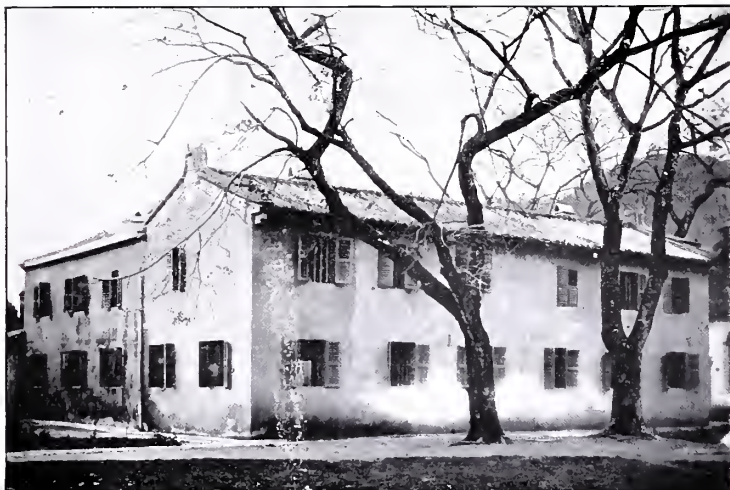
WUKINGFU HIGH SCHOOL: MAIN BUILDING.
